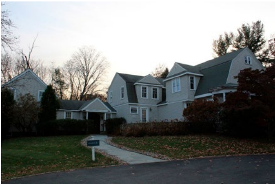
The three stories FARIL lab building, outside view.
